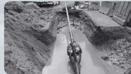
Horizontal Directional Drilling
