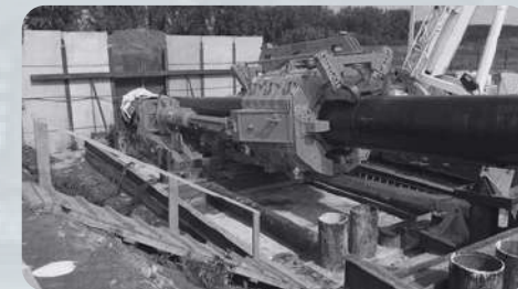
Horizontal Directional Drilling
